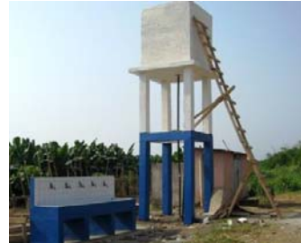
Boyer Water Tower and Hand Wash Station, Ivory Coast
