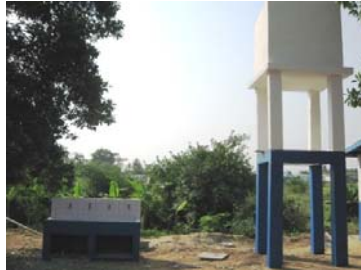
Lagonda Water Tower and Hand Wash Station, Ivory Coast
